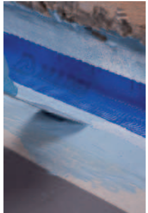
Application of Mapeband to a wall-floor joint with Mapelastiq AquaDefense
