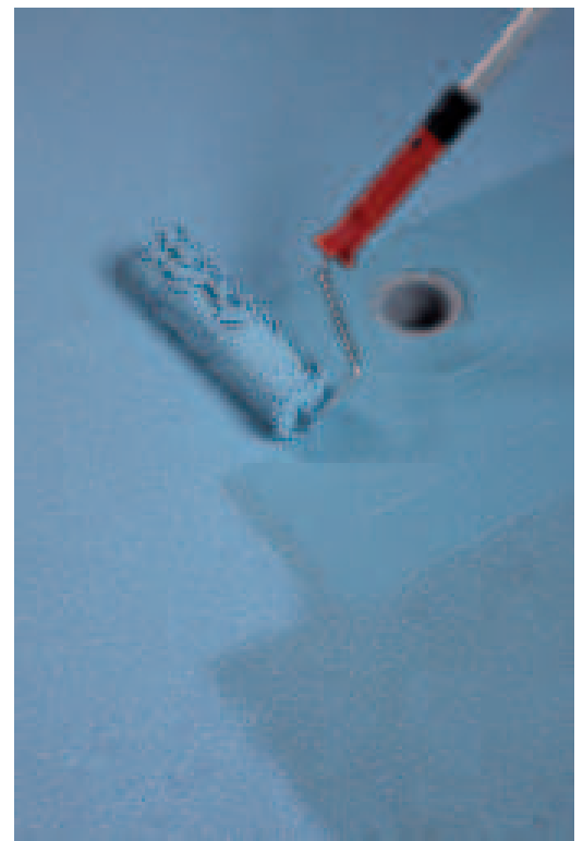
Application of the second coat of Mapelastiq AquaDefense
